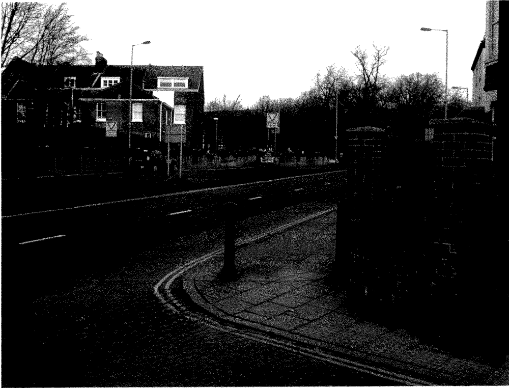
Poor visibility splay at entrance to Lyon Street
